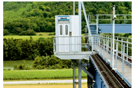
↑ Access – stairs, platforms, ladders and elevator
