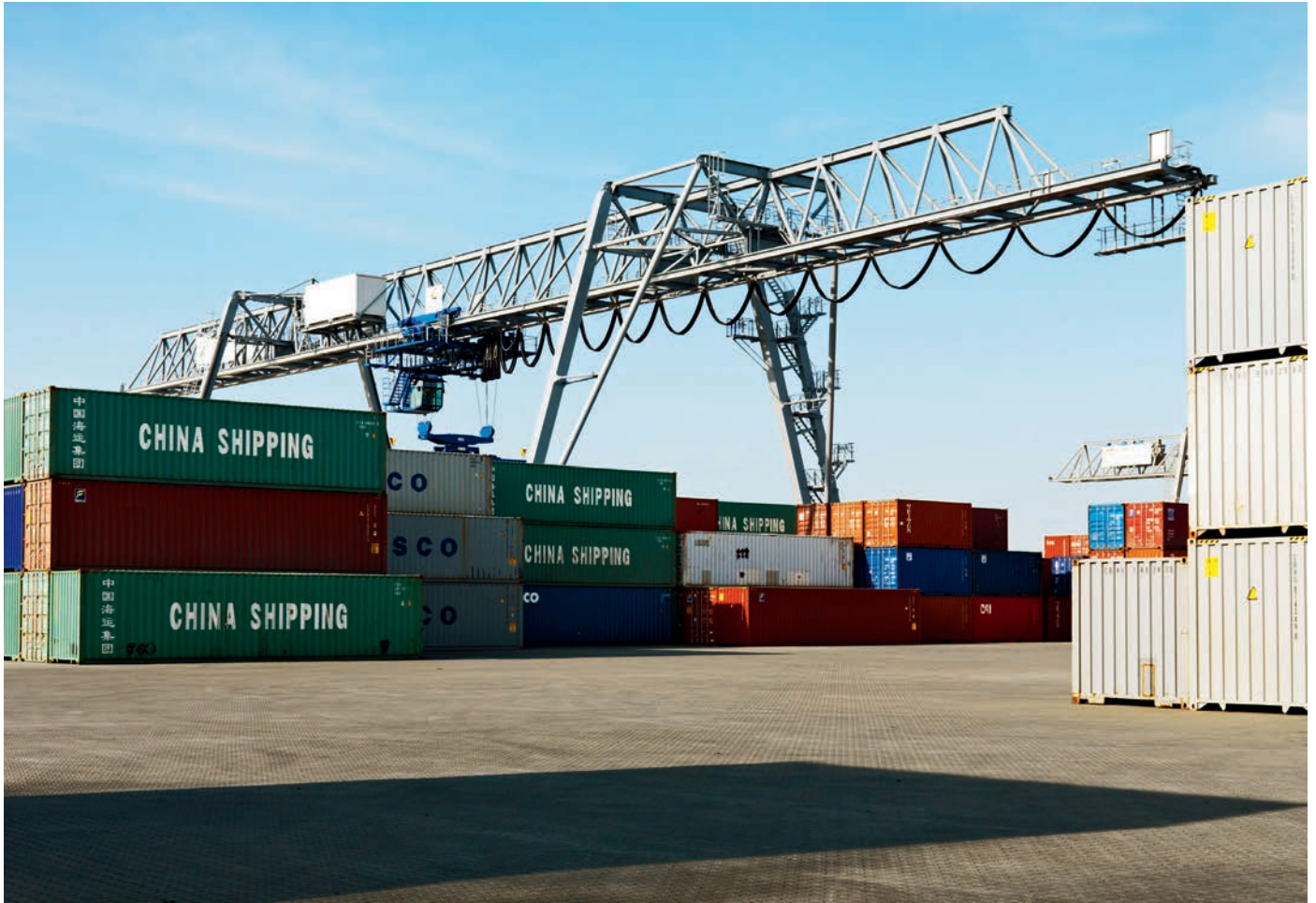
↑ Inclination of the gantry supports
